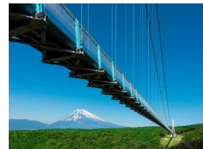
Mishima Skywalk (photo supplied by Fujico Corporation)
