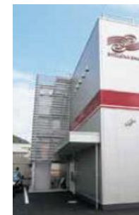
[Outdoor upstairs to rooftop]
