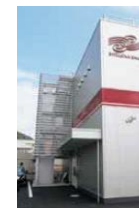
[Outdoor upstairs to rooftop]
